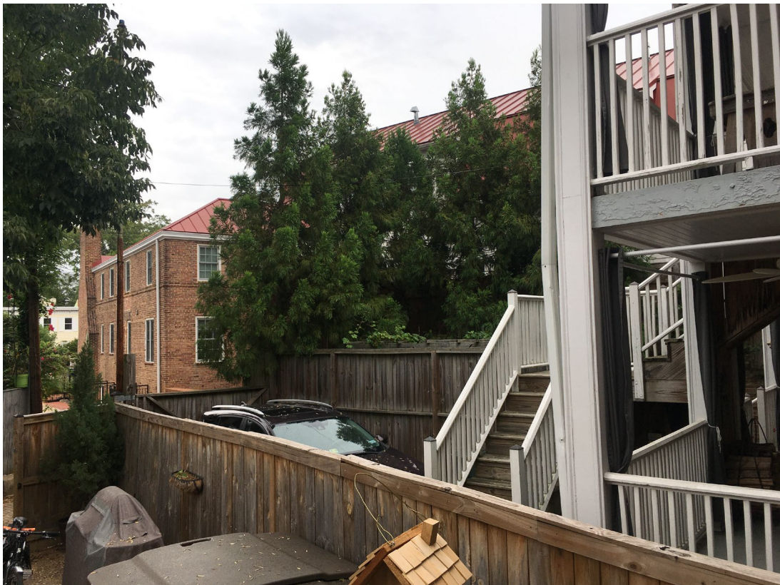
VIEW FROM REAR YARD LOOKING NORTHEAST
