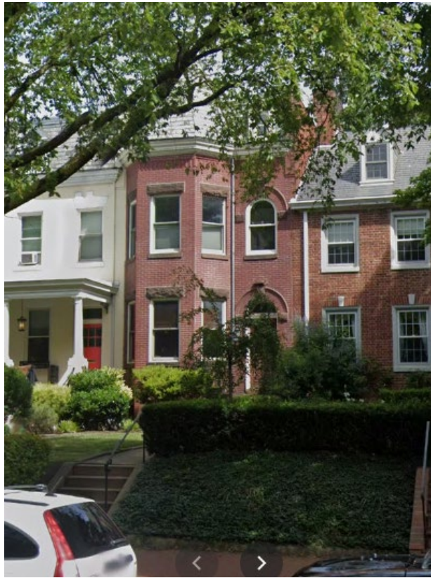
EXISTING FRONT FACADE
