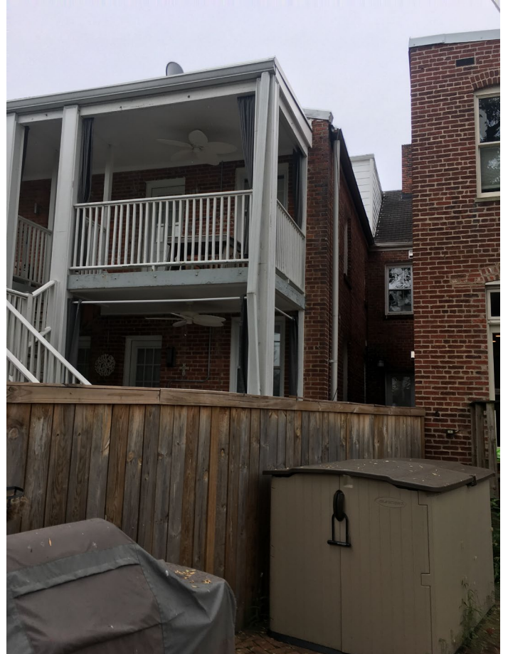
FROM REAR YARD TOWARD 616 S. CAROLINA AVE SE
