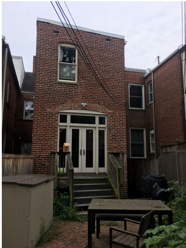
EXISTING REAR FACADE
