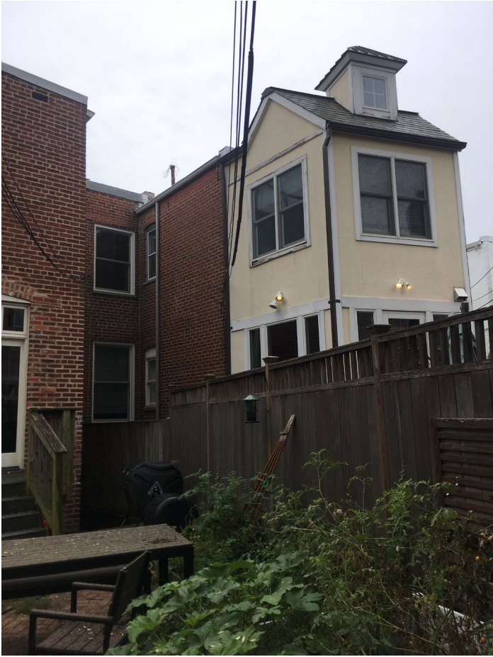
FROM REAR YARD TOWARD 608 S. CAROLINA AVE SE
